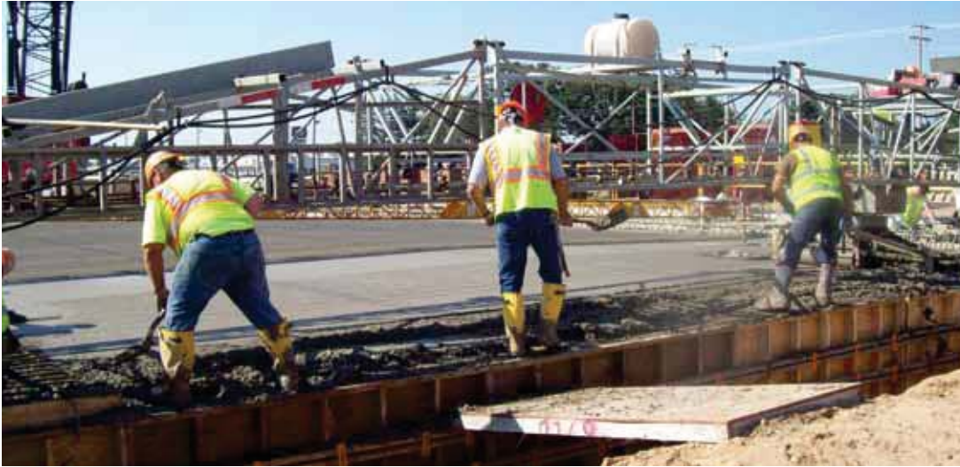
Workers pour a concrete structure on Koeller Street in Oshkosh
